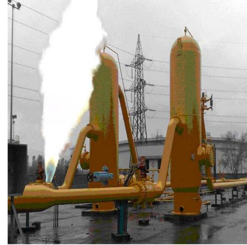
The jet fire is a effect of a leakage ignited from a pressurized equipment like flanges, cracked pipe work or vessel, fittings damaged, and generating high heat fluxes over 300 kW/m2, flame temperature of 1350 ° C, according different sources (HSE, SINTEF, etc.), with irreversible and domino effect on structures attacked by the jet fire.
